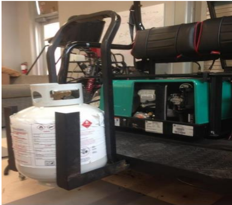
Figure 9. Propane tank mount and location
